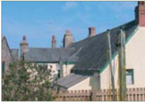
Bitumen coating in Rectory Lane
