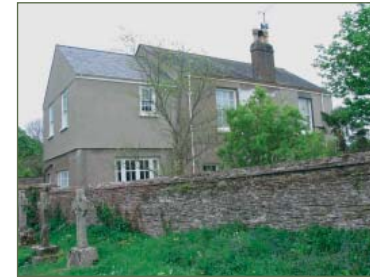
Former meeting Room
