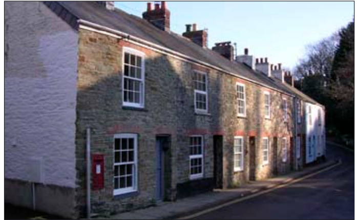
Shadycombe Lane - row of cottages
