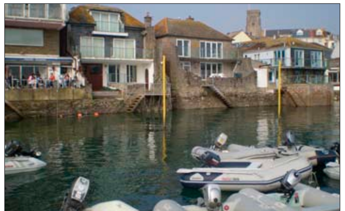
Balconies, railings and patio doors on converted warehouses
