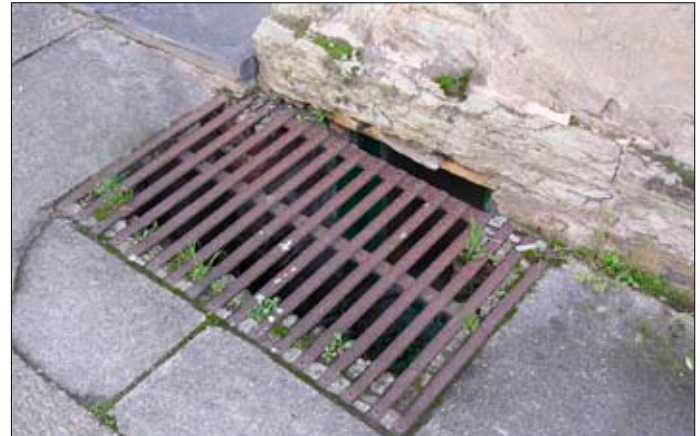
Church Street - grille to pavement for basement light
