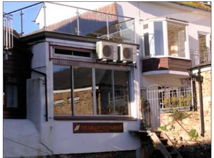
Ugly air con, patio doors to waterfront inlet
