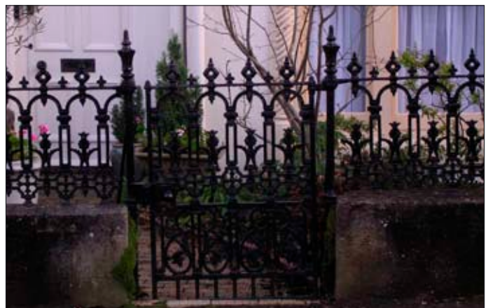
Devon Road - cast iron gates and railings to front gardens
