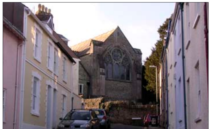
View up Church Street to east end of the church
