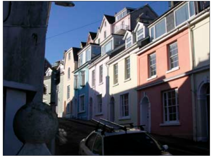
Courtenay Street. View of dormers to front elevations
