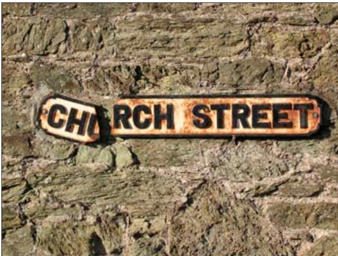
Historic street name sign - broken
