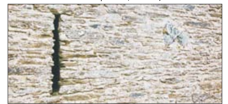
While thin-bedded stone is the dominant walling material, bringing much harmony to the street scene (above), a great many houses and cottages in the Area are colour washed, either directly onto the stone to preserve its undulating, rustic charm, or over a render coat to present what many an 18 th or 19 th century owner thought a more dignified and 'proper' appearance (see Jaspers, far left).
