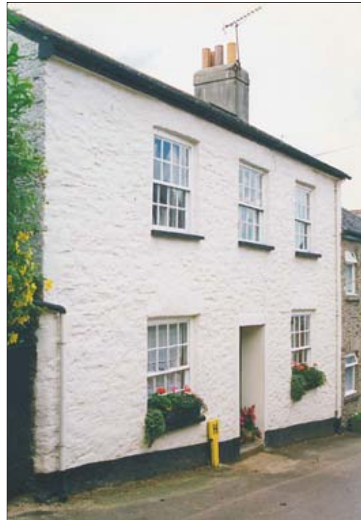
While the architectural quality of the Old Rectory isn't repeated, a few other houses in the Area illustrate the more formalised 'polite' designs of the 18 th and 19 th centuries. Whether original or 'planted' (onto an older fabric) the most pleasing and characterful are those like Maynards which retain their authentic painted timber windows and doors (above). The majority of houses and cottages, however, have a less formal, vernacular, style characterised mainly by 'irregularities' in the arrangement, size and style of their windows. Berries Farm (left) is an example. It examples too a plain, flush ridge to its thatched roof (not an ornamental, block-cut one) which respects local tradition.
