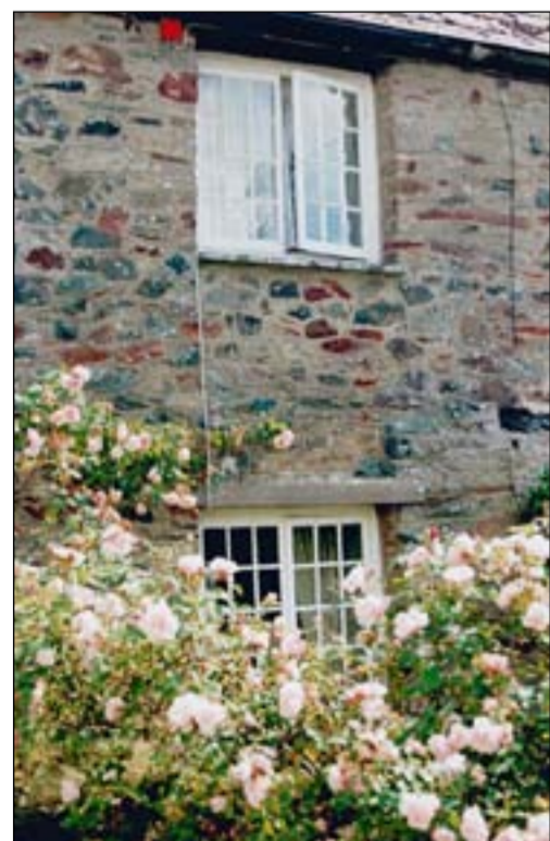
This small-paned window pattern is typical of the estate cottages created through conversion
