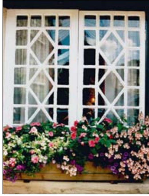
One of the many painted timber 'lattice' casement windows that signal estate construction
