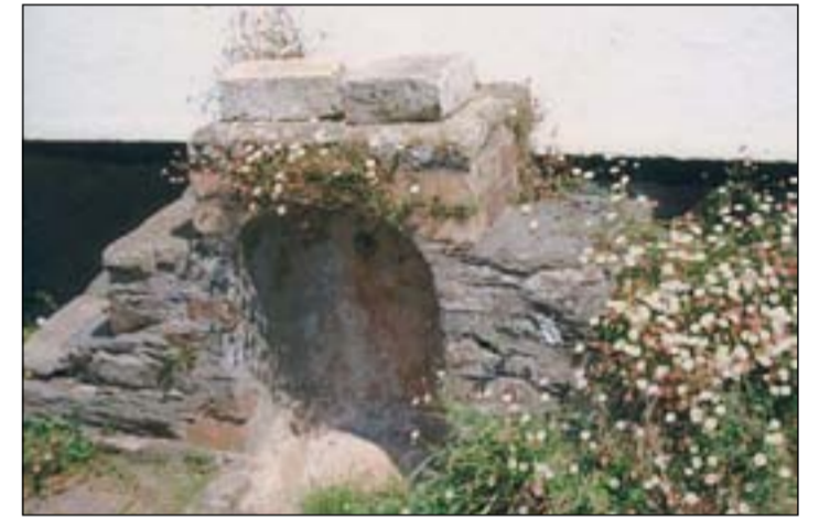
The combined water supply and mounting block against the wall of the Durant's coach house
