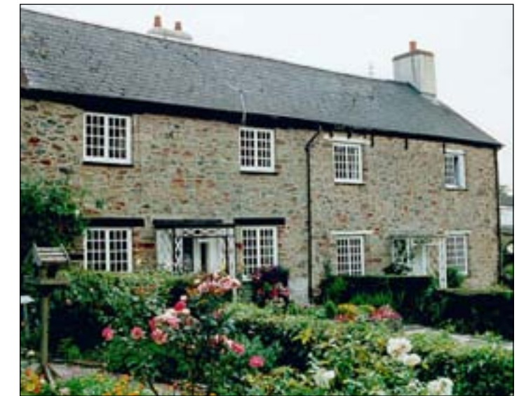
Not all the estate cottages were newly built. These look to be 19 th century but some earlier features confirm they were converted from a former farmhouse and shippen range
