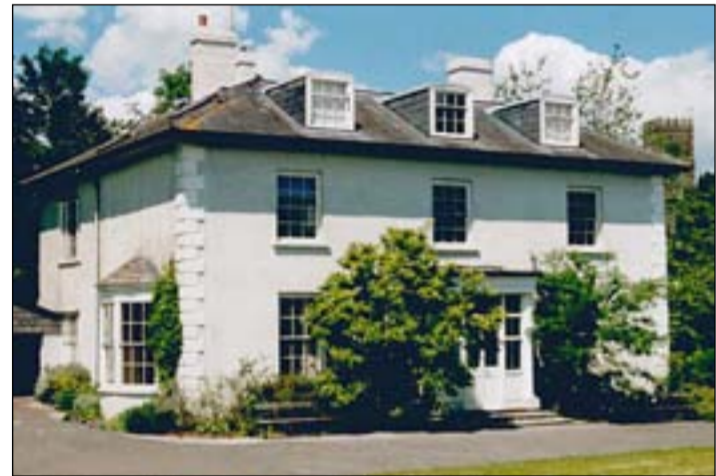
Here in its private setting, Ashprington House occupies spacious grounds characteristic of its age and status. The dormers aren't original but were added to the roof shortly after the house was reduced from 3 to 2 storey in the mid 20C
