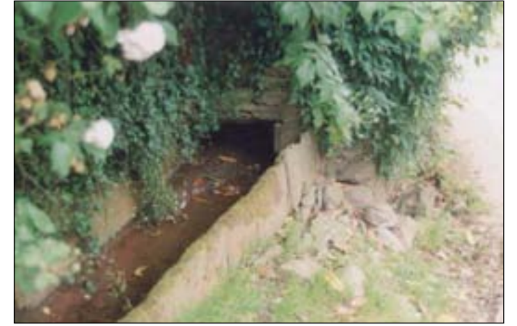
A section of the rather ingenious drainage channelling
